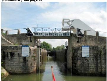
The locks were many and small, generally accommodating no more than two boats, end to end. All of the locks were automatic, triggered by a cord hanging in the middle. You approach the lock, wait for it to open and give you the green light and enter the lock. It closes behind you, you climb the ladder on the side, pull the cord and the pumps start to run.
